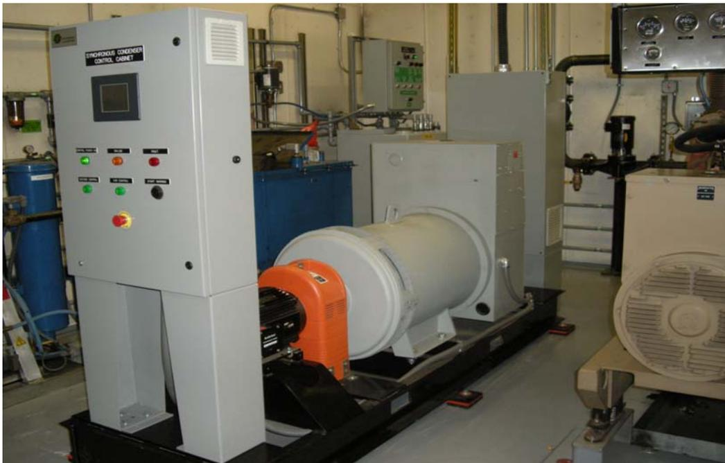
power (kVAR) output. The synchronous condenser is thus a continuous variable source/sink of reactive power.
